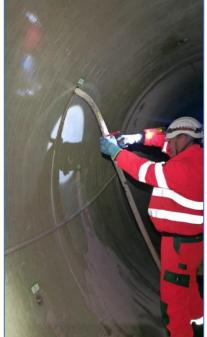
Figure 13. Grout injection phase through valves
