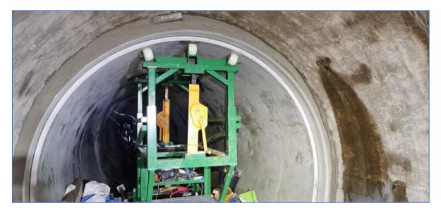
Figure 10. Mortar sealing
