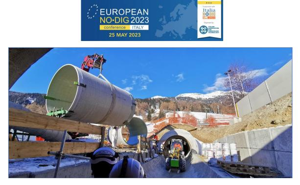
Figure 7. Transport and insertion of GRP pipes in tunnels
