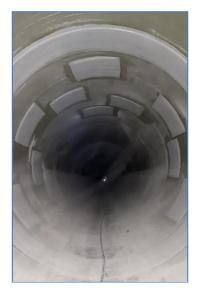
Figure 14. Laminated joints and nipples
