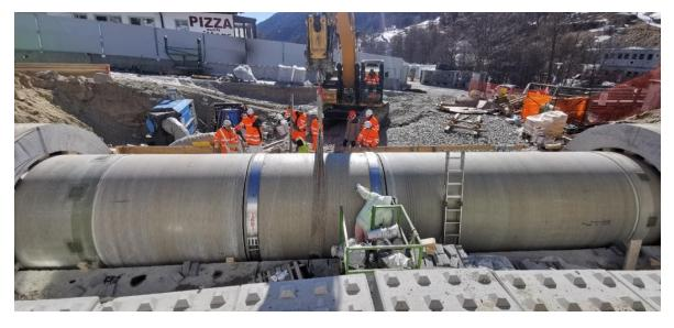
Figure 9. Joint connection system STRAUB OPEN FLEX3 – Last GRP piece
